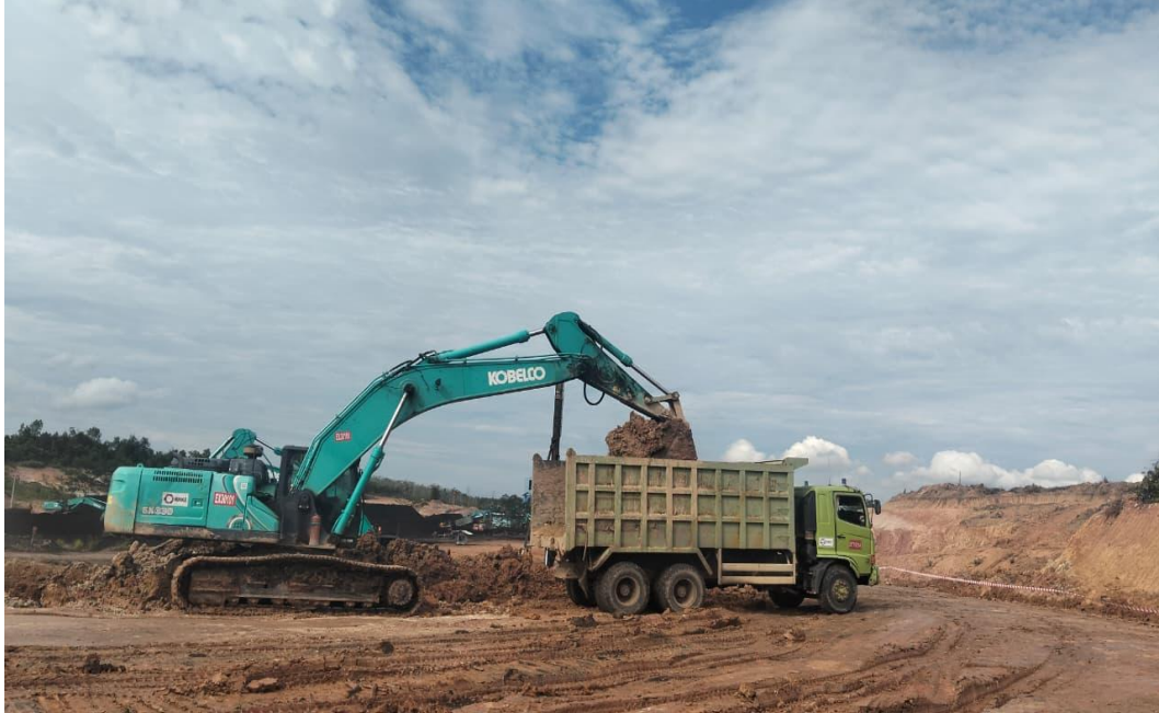
Gambar C.2 Loading Top Soil ke Dump Truck
