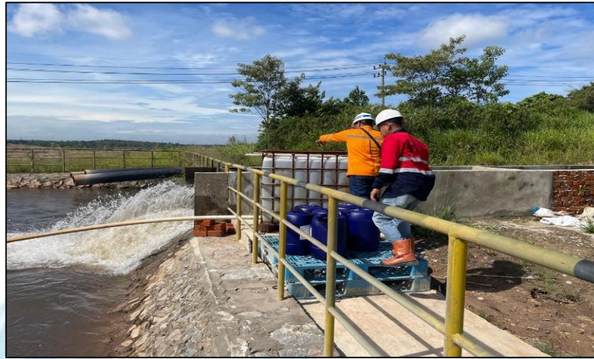
Gambar 4.3 Pemberian Chemical Coagulant
