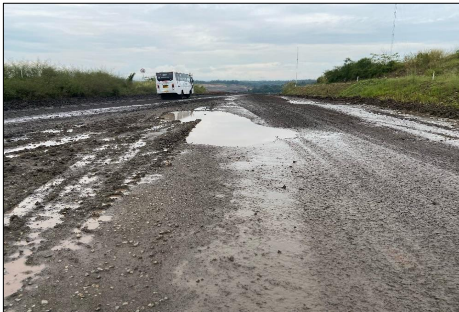
Gambar 3.5 Potholes Jalan AWR
