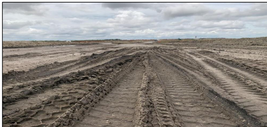
Gambar 3.4 Rutting Jalan AWR
