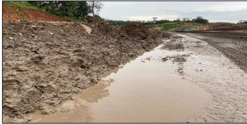
Gambar 3.6 Inadequate Roadside Drainage Jalan AWR
