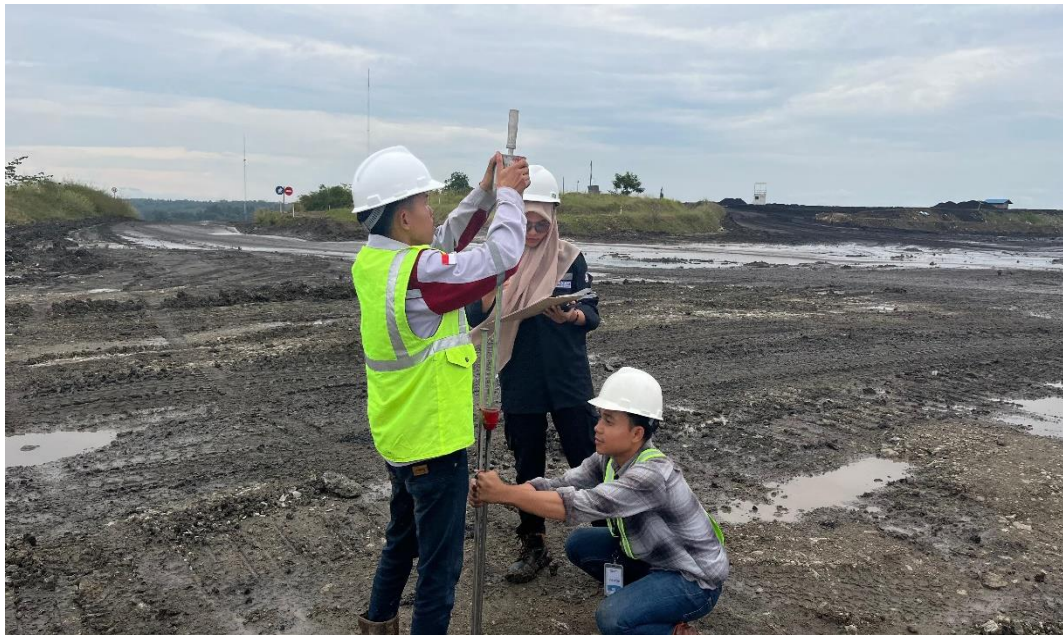
Gambar K.2: Uji Dynamic Cone Penetrometer
