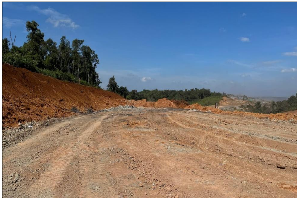
Gambar 3.1 Improper Cross Section Jalan AWR
