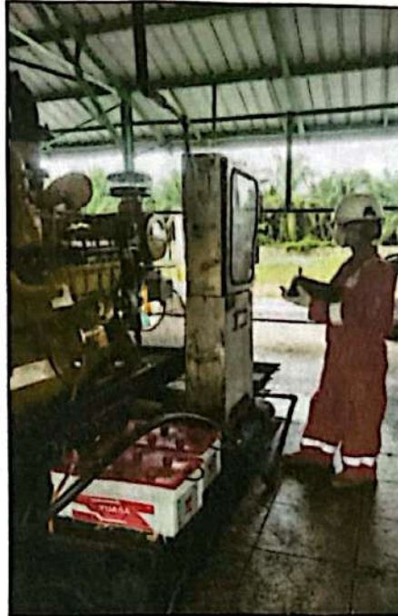
Gambar C.1 Pengecekan Tekanan Gas Engine
