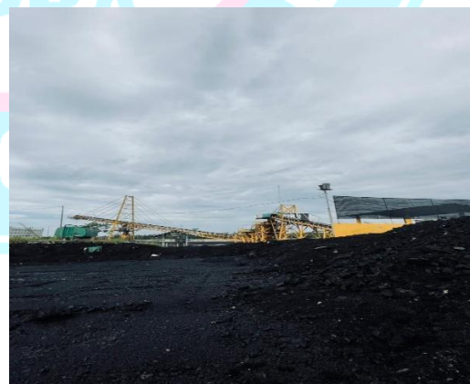
Gambar F.6 Area Crusher B
