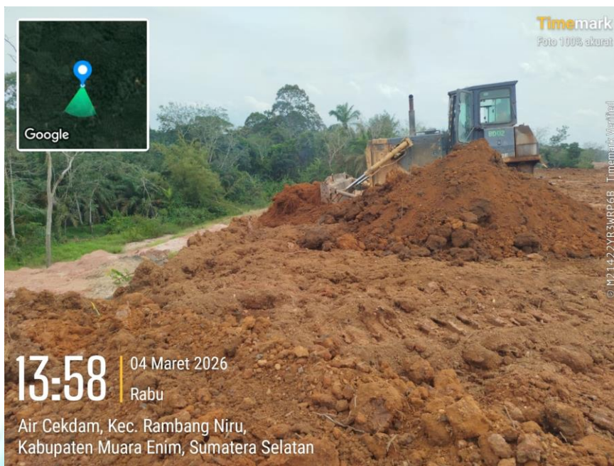
Gambar A. 3 Pushing and Filling Material Top Soil
