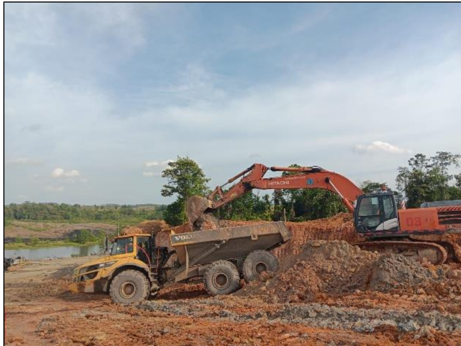
Gambar 2.8 Kegiatan Pengupasan Top Soil
